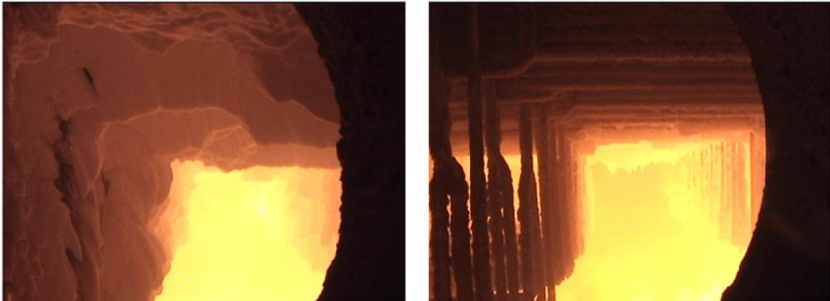
**Figure 5 Improved boiler operation before (left) and after optimization**
